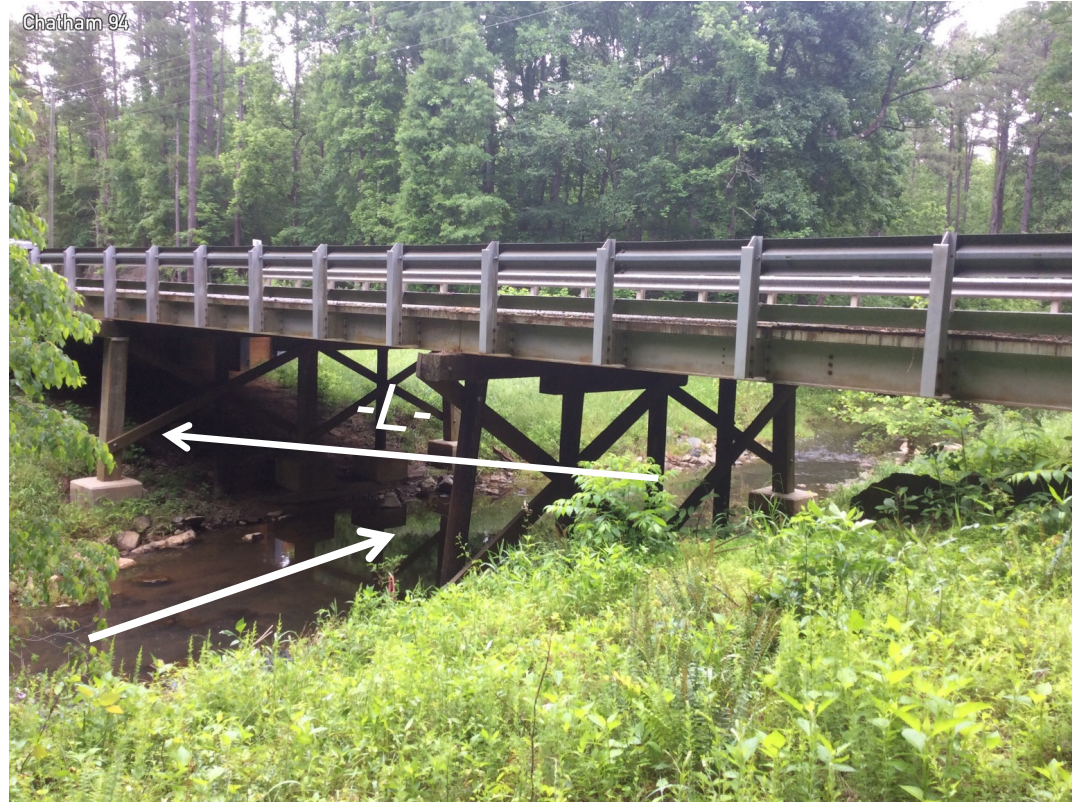
BRIDGE NO. 94 FACING NORTH EAST
