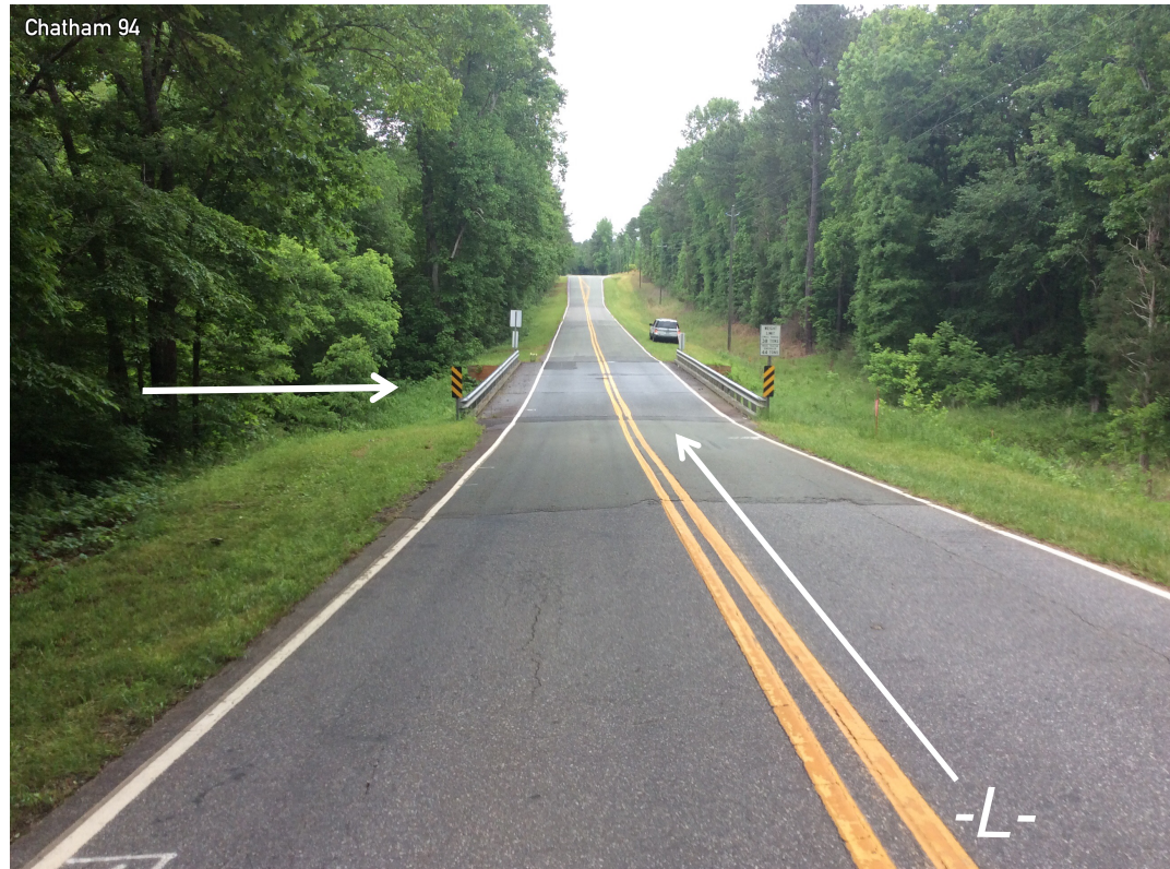
BRIDGE NO. 94 FACING NORTH - AHEAD STATION
