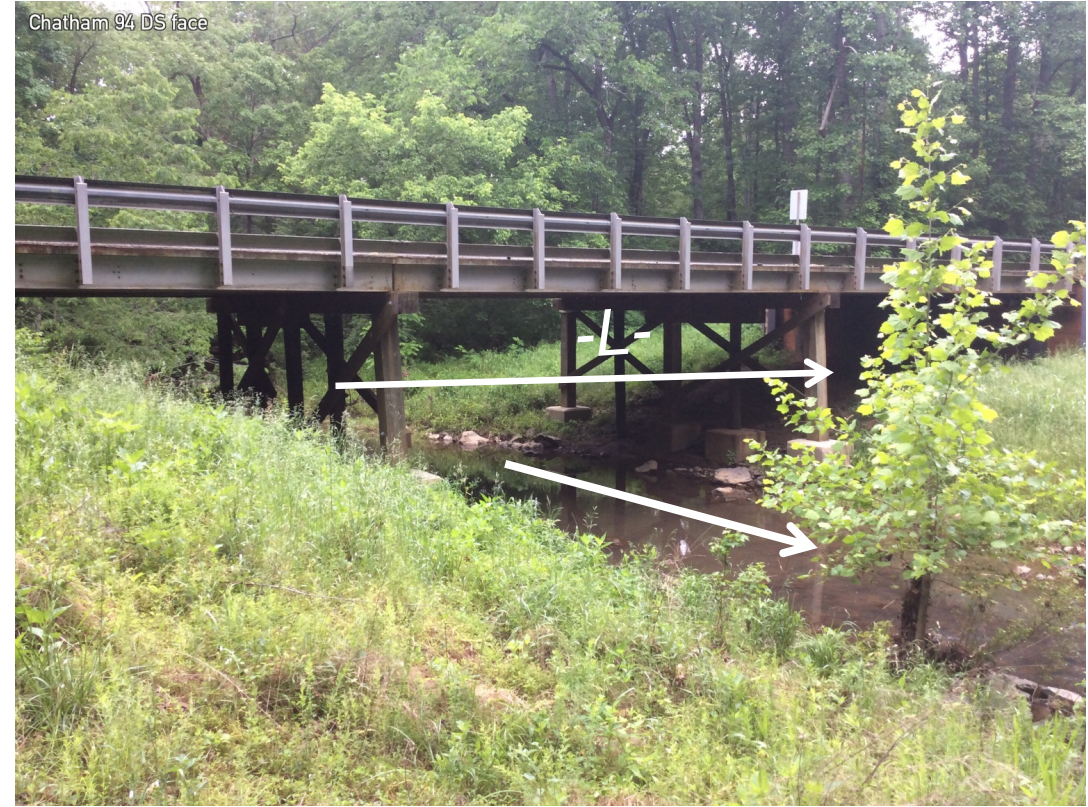
BRIDGE NO. 94 FACING NORTH WEST
