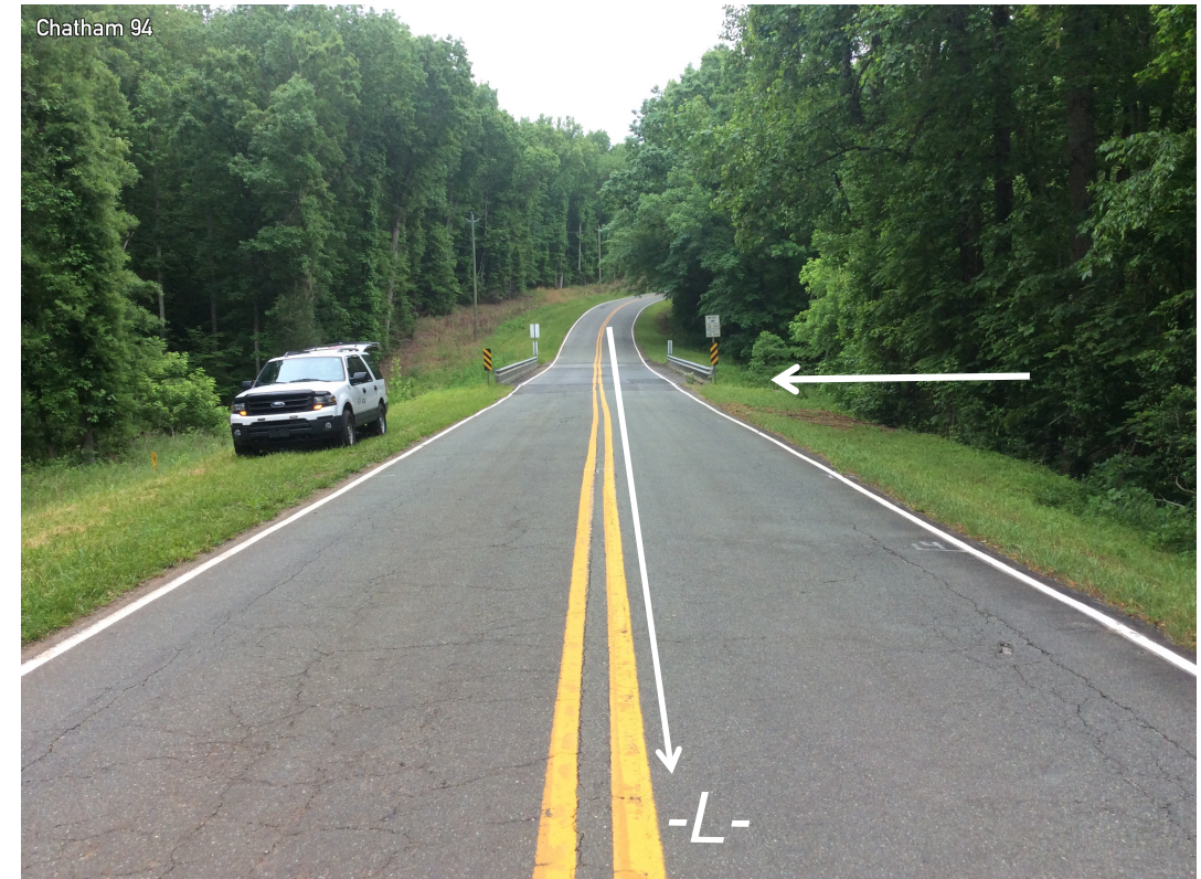
BRIDGE NO. 94 FACING SOUTH - BACK STATION
